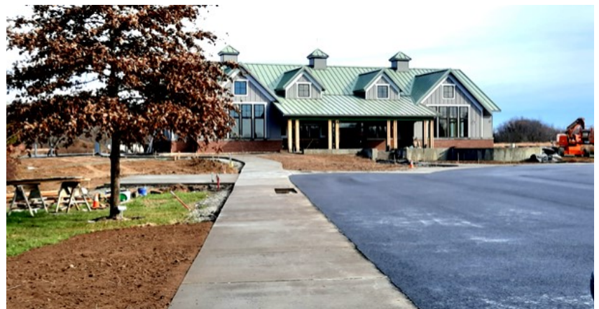
The new Visitor Center in progress Photo by T. Lewis
